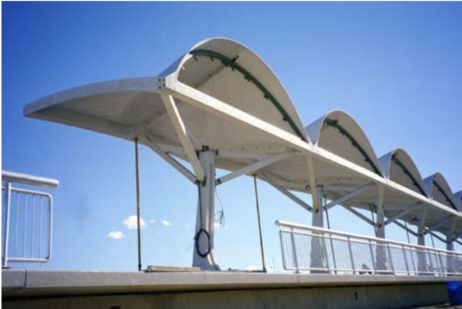
Fig. 3 Structure of Shawnessy Light Rail Transit Station
