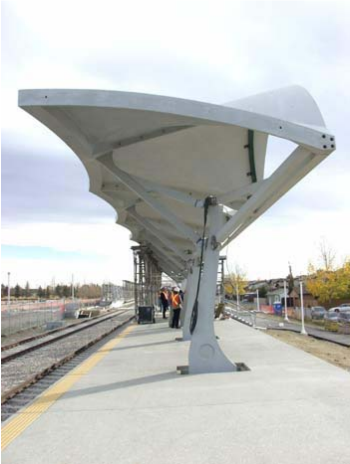
Fig. 4 Structure of Shawnessy Light Rail Transit Station
