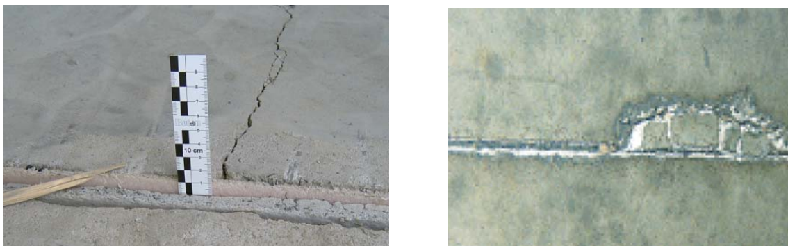
Fig. 1 Curling (left), damage near joint due to traffic
