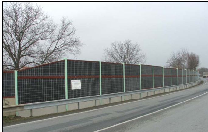
Fig. 5 Absorptive sound protection wall, Modřice
