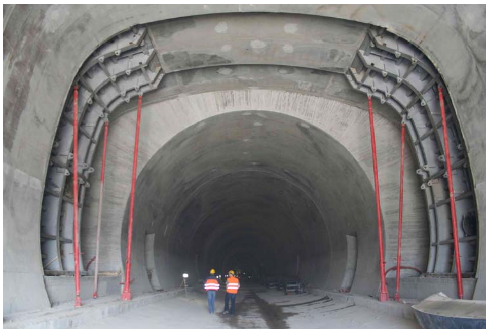
Fig. 1 The New Connection railway tunnel
