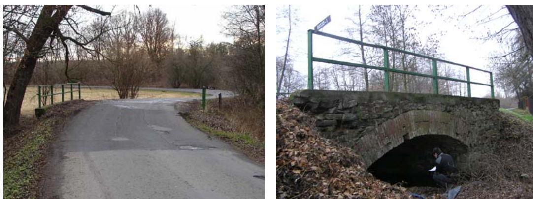
Fig. 5 Convenient object for installation of reinforcement from the road surface, Czech Republic.
