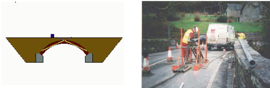
Fig. 4 Typical anchor positions and installation of reinforcement from the road surface.
