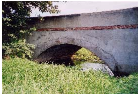
Fig. 3 A Lined Bridge, England
