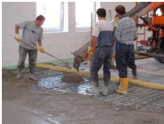
Fig. 3 Repair layer. The mesh could be placed parallel to pouring of the concrete
