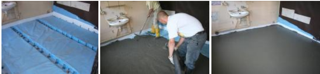
Fig. 10 Arranged ceiling before casting (left), casting of SFRLWC (middle), finished timber-concrete-composite ceiling
