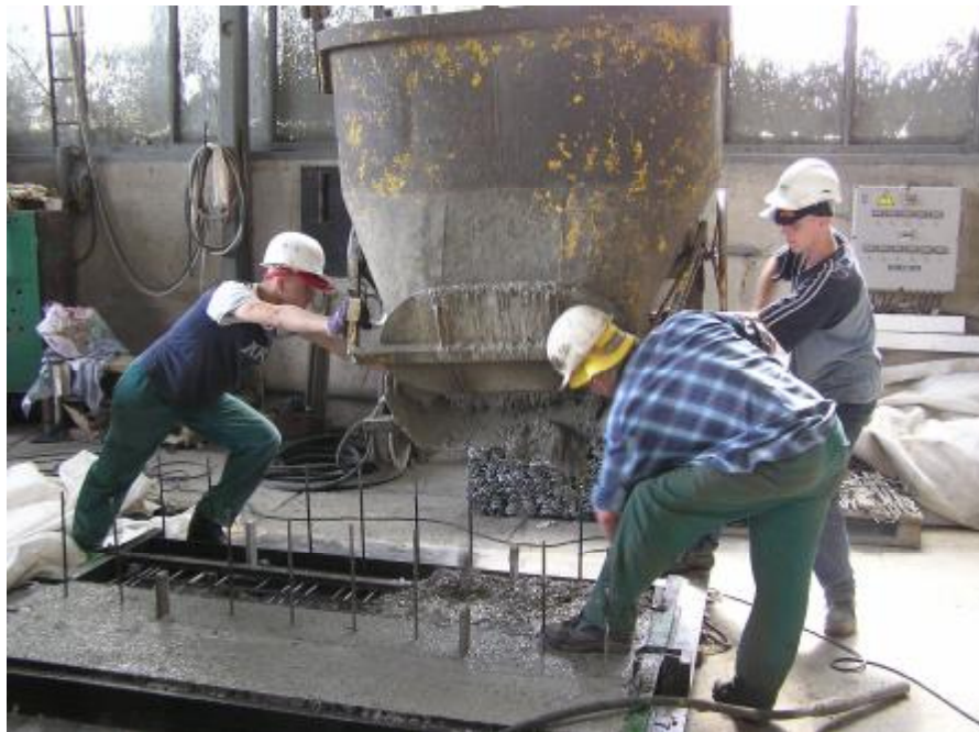
Fig. 3 Placing concrete into the form
