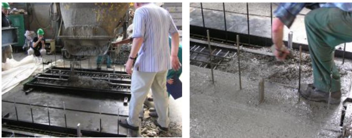
Fig. 1 and Fig. 2 Casting of fiber concrete member
