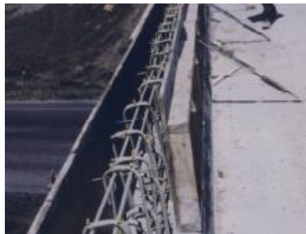
Fig. 6 Steel reinforced jersey barrier
