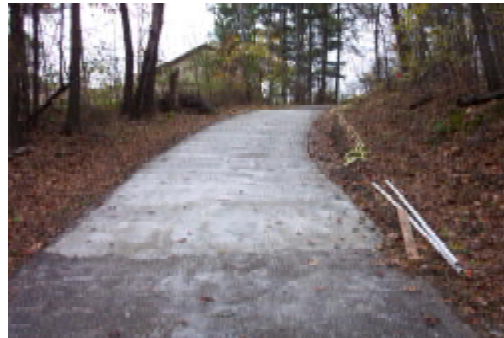
Fig. 7 UTW residential driveway
