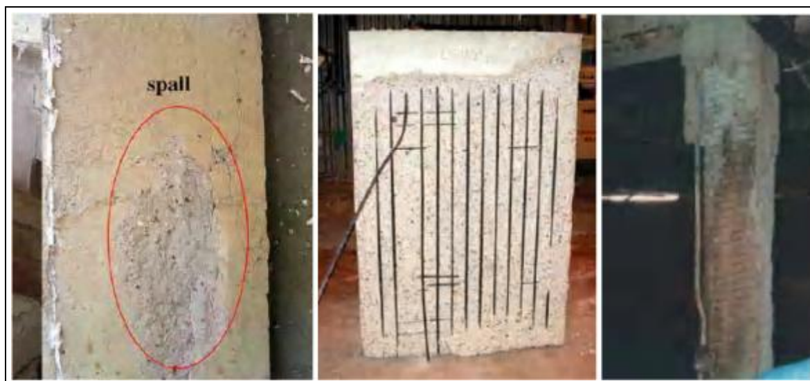
Fig. 1 Spalling of concrete after high temperature exposition [3, 11]
