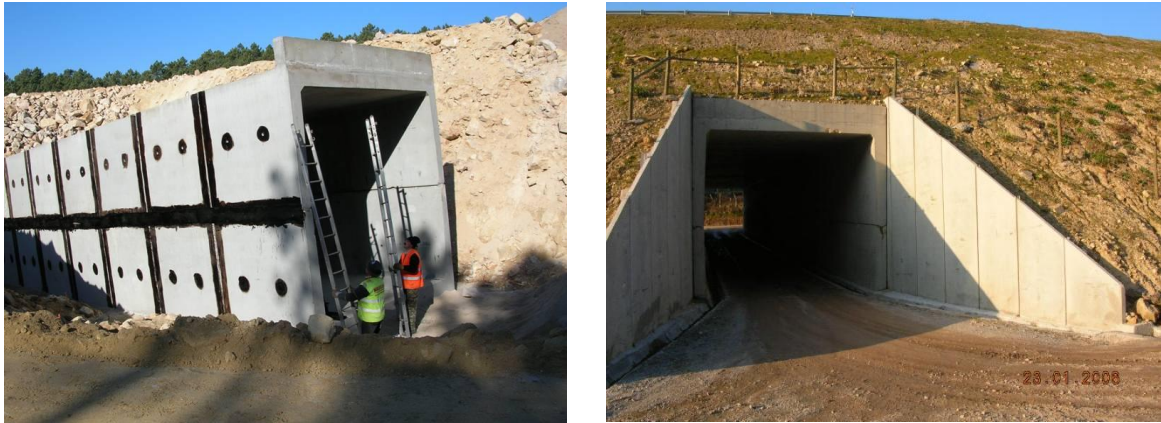
Fig. 28: Examples of application of box-culvert.
