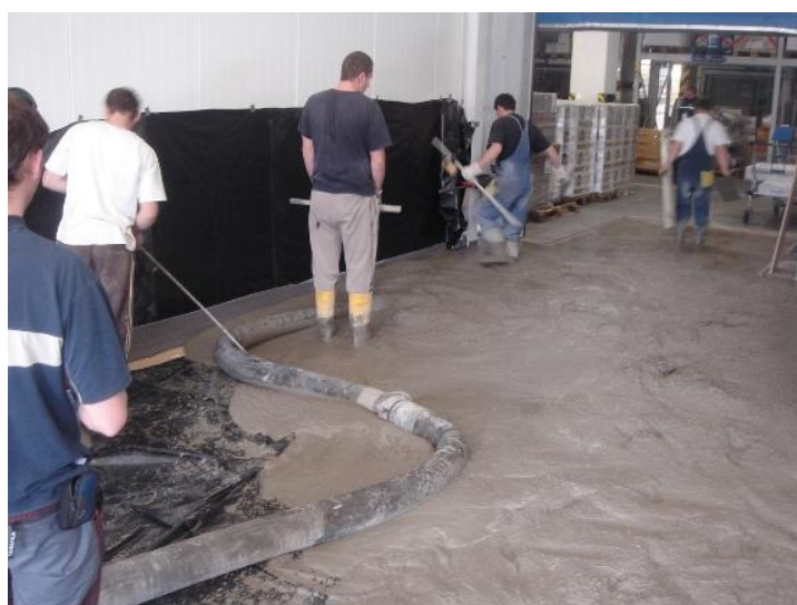
Fig. 1: Fresh concrete working-up
