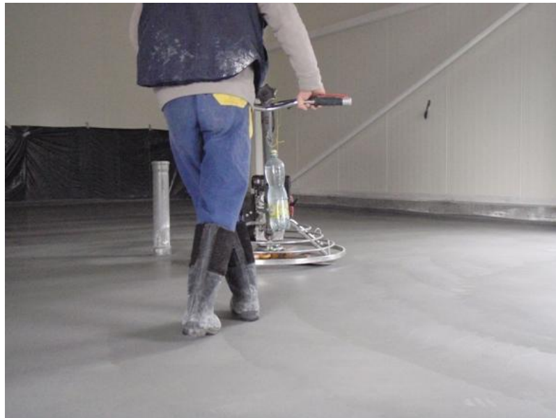
Fig. 2: Surface treatment by rotary iron
