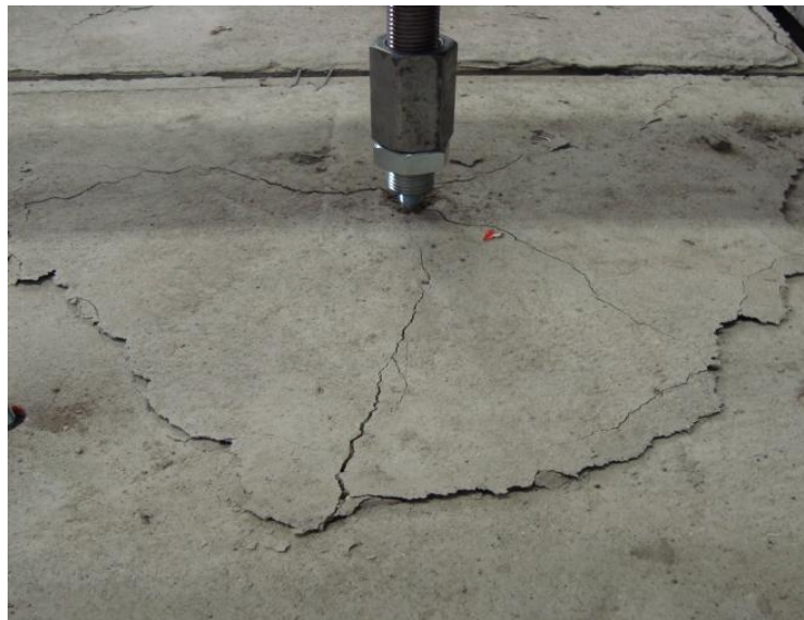
Fig. 8: Pull out failure
