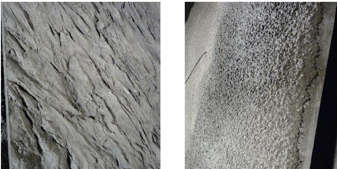
Fig. 1 Artificial rock wall before (left) and after spraying of concrete (right).
