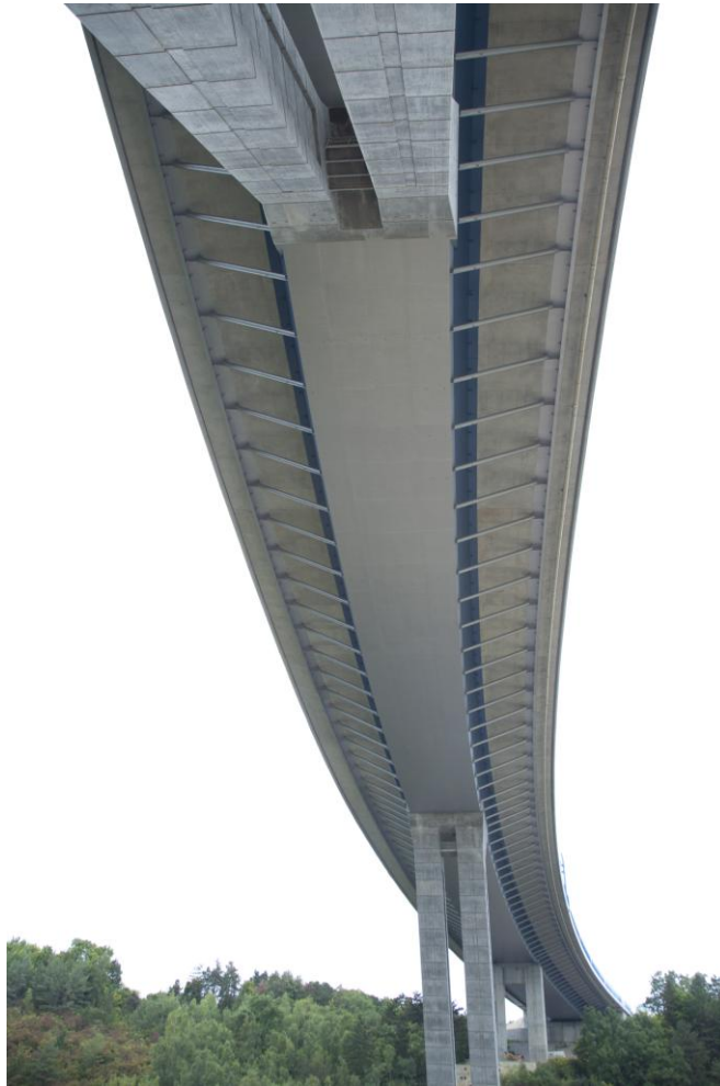
Fig. 3: Bottom view of bridge
