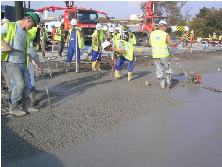
Fig. 5: General view of the lying and compacting of concrete with PP microfiber Fibrax 12
