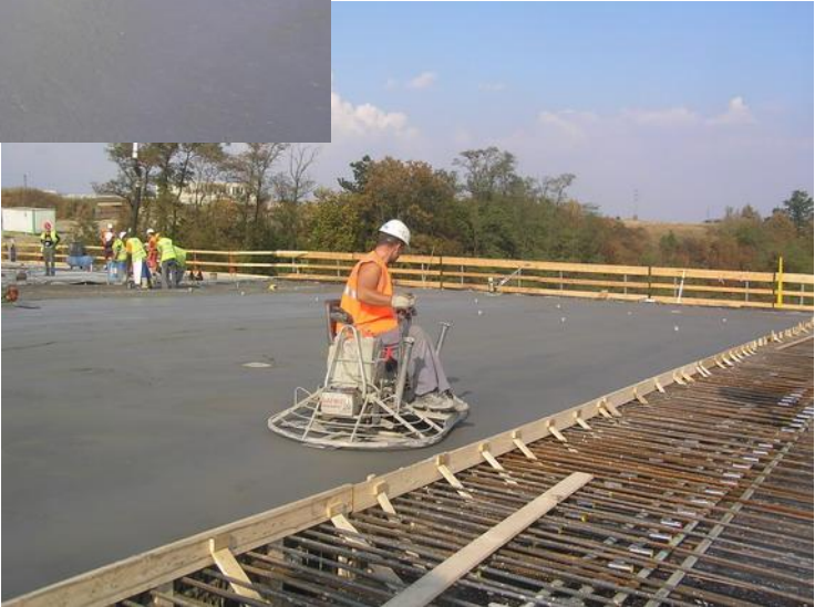
Fig. 6: General view of surface finishing of concrete with PP microfiber Fibrax 12
