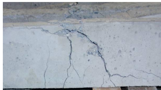
Crushing of concrete
