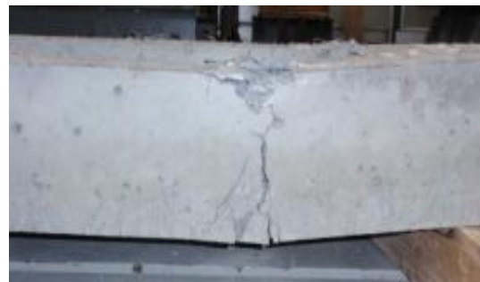
Flexural cracking failure
