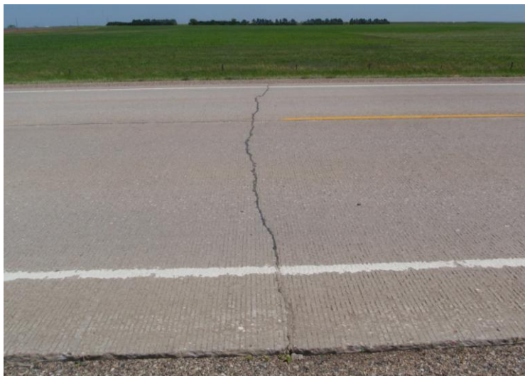
Fig. 1: Full depth FRC pavement crack
