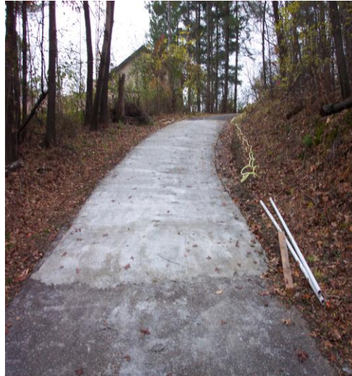
Fig. 2: First of five FRC overlay asphalt placements
