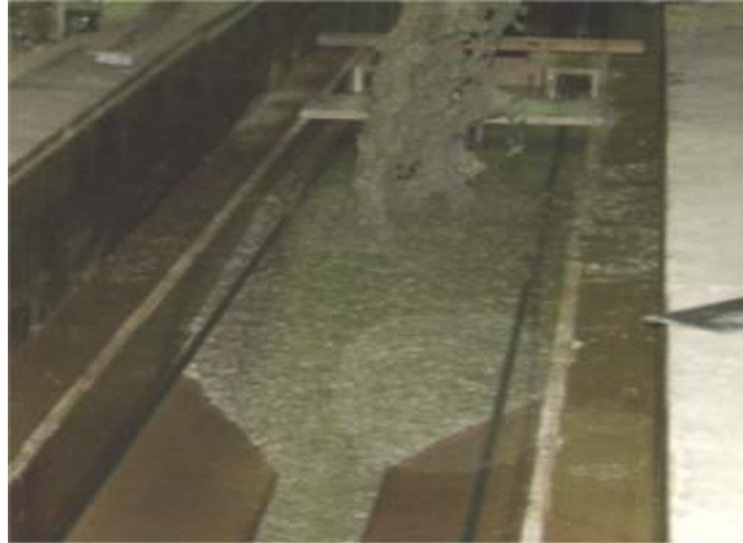
Fig. 4: The concrete shown flowing from the discharge point in mid span to end of the beam
