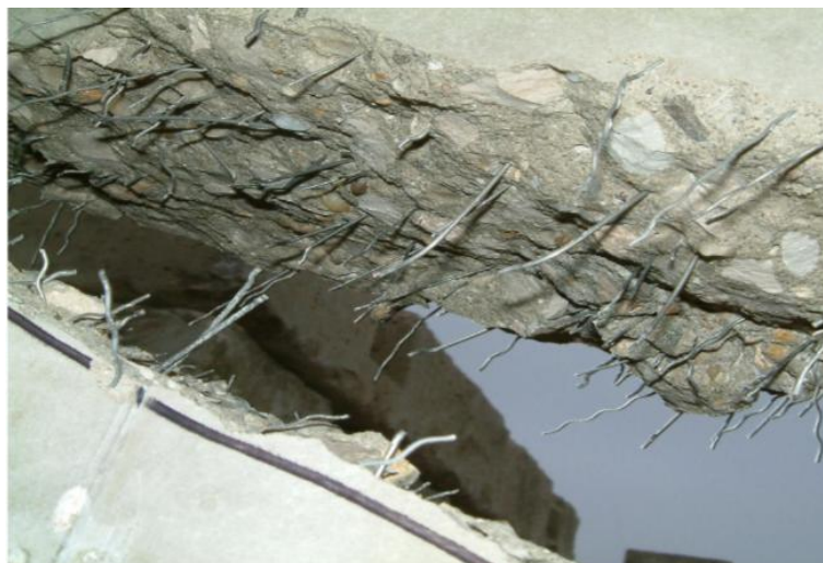
Fig. 9: Fracture surface of the experimental girder
