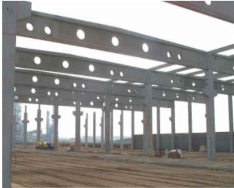
Fig. 11: PM Leuna under construction
