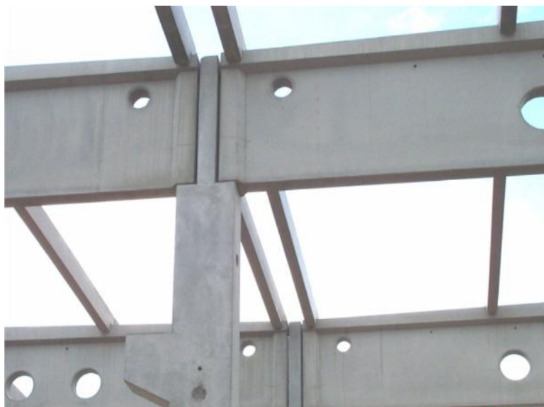
Fig.12: roof trusses and purlins; the spacing between the trusses is 10 meters
