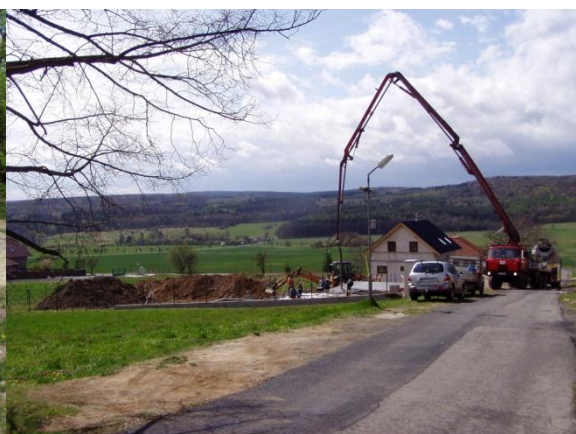
Fig. 8: Placing concrete bed-slab in Kublov
