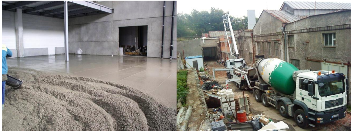
Fig. 11: Placing FLOORCRETE – enlargement of airport halls at the Mosnov airport
