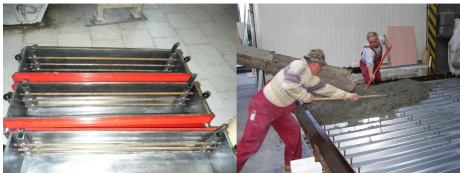
Fig. 9: Prepared moulds with reinforcement before STEELCRETE was placed
