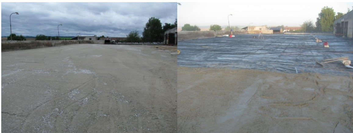
Figs. 9 and 10: Preparation of sub-base
