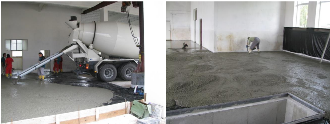
Figs.1 and 2: Casting of concrete
