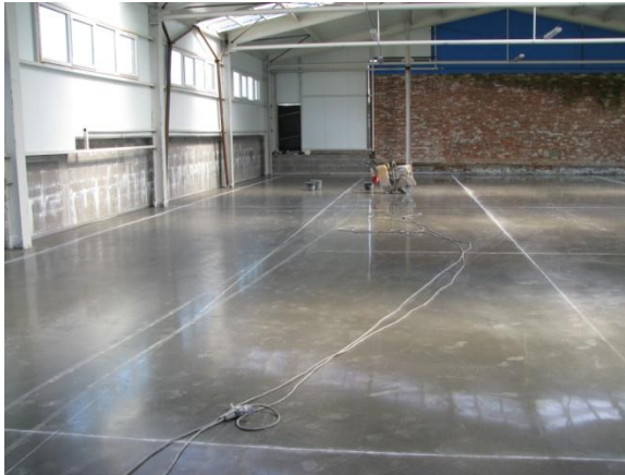
Fig. 7: Finishing of slab – cutting of joints
