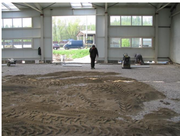
Fig. 5: Preparation of sub-base
