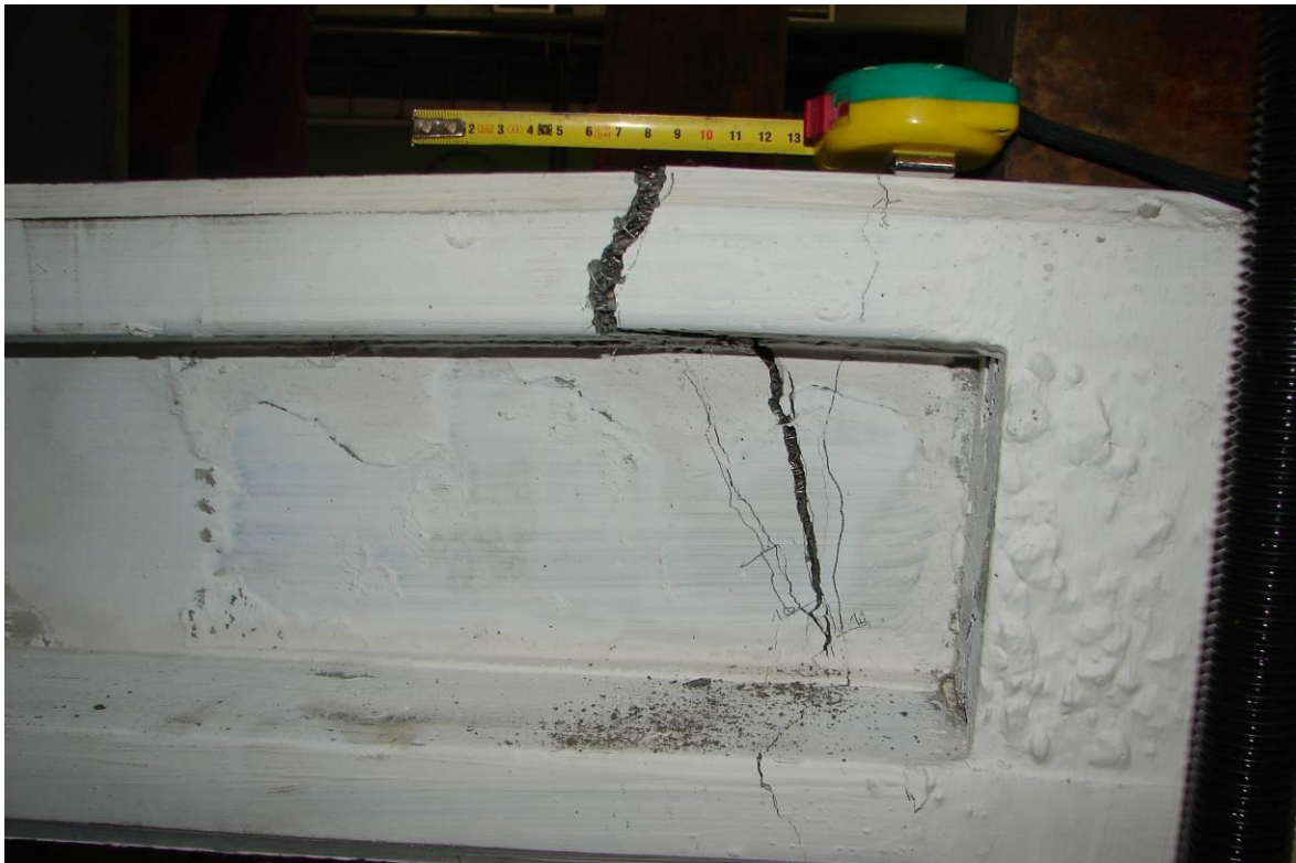
Fig. 3: The failure of cantilever beam at fixed point
