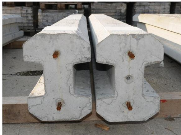
Fig. 2: End section of a prestressed precast pier
