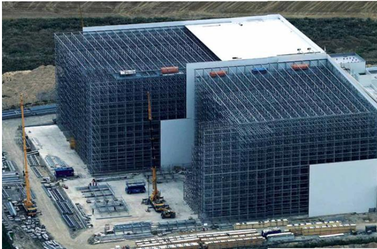
Fig. 9: Illustration of a typical CladRack system
