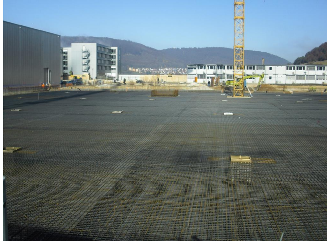
Fig. 8: Structural floor of an extremely high demanding building: Combined solution
