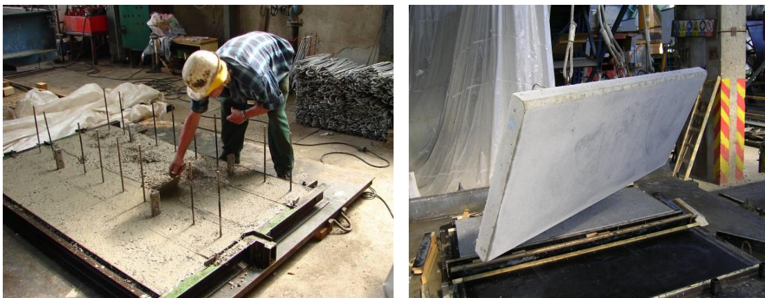
Fig. 1: Casting of FRC member; (b) lifting from the formwork
