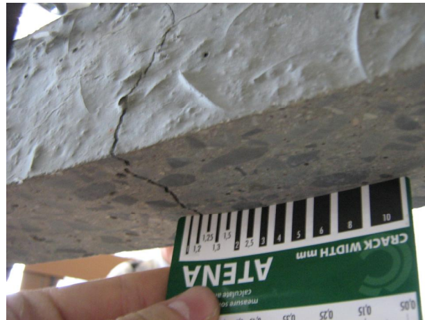
Fig. 4: Control measuring of the crack width after three-point bending test
