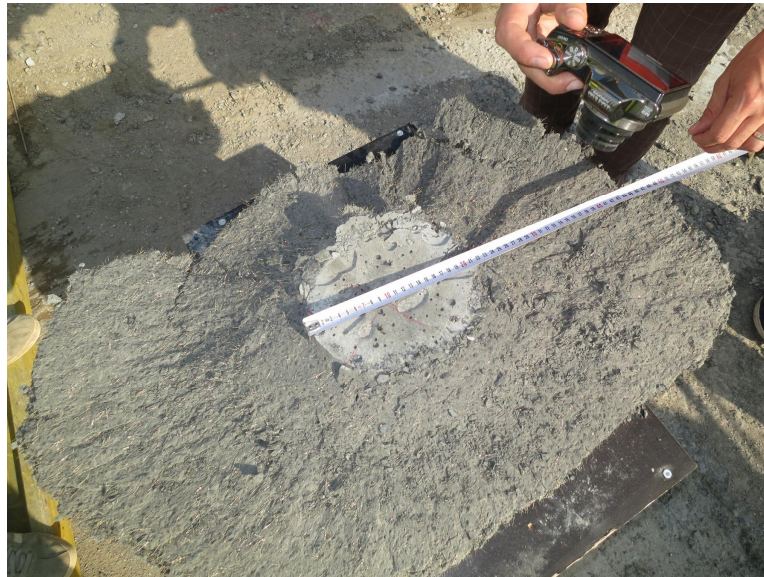
Fig. 9: Failure of the slab – detached concrete
