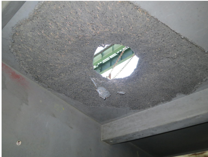
Fig. 8: Failure of the slab from the bottom
