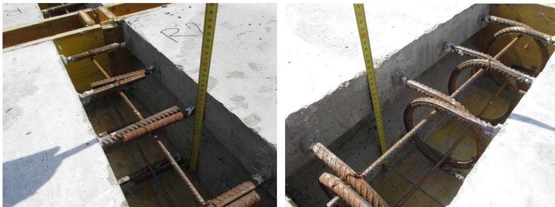
Fig. 6: Straight bars in UHPC joint (type R) and bars in the loop (type S)
