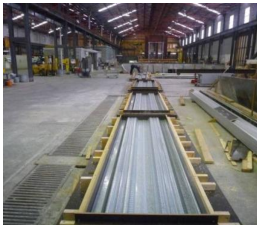
Fig. 2: Formwork and slab immediately after casting.
