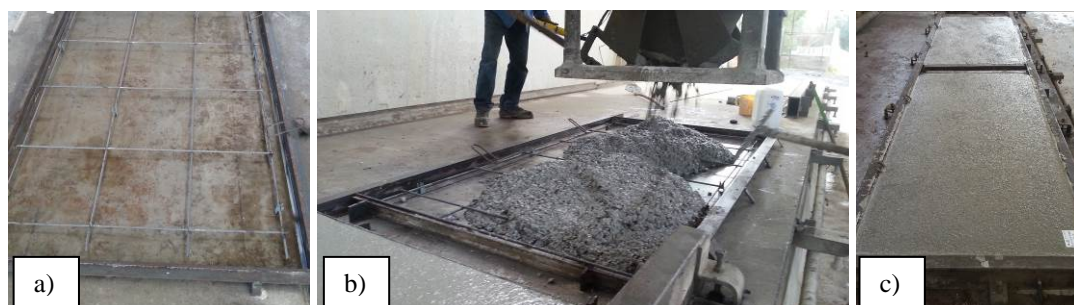
Fig. 5: Production of the panels: a) steel moulds; b) casting; c) prototypes
