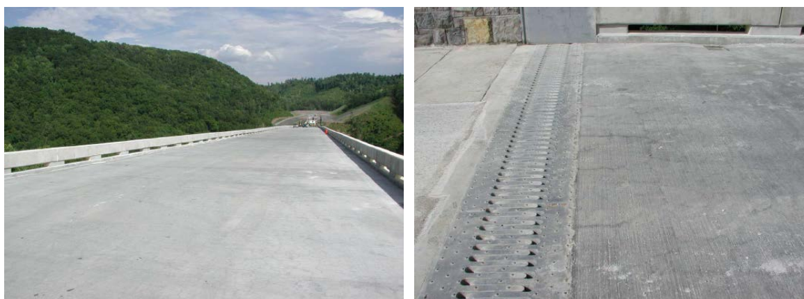
Fig. 1: Exposed concrete pavement on bridge over Wilson Creek, Montgomery County, Virginia, USA [1].
