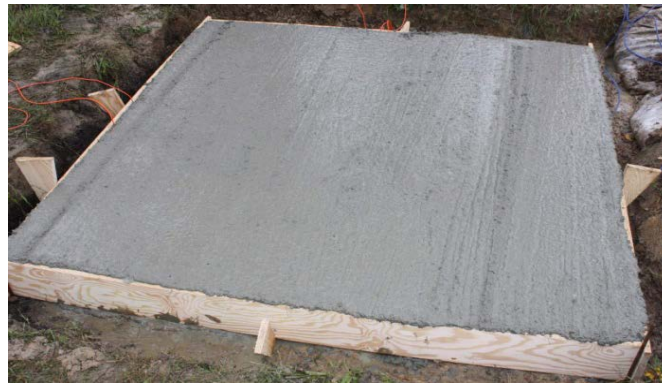
Fig. 1: Casting of the fibre concrete slab
