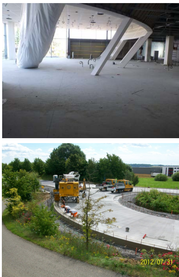
Fig. 8: Self-leveling screed project for a high-end automobile dealership, France (above) and Roundabout road K 1060/1013 in Renningen, Germany (below)
