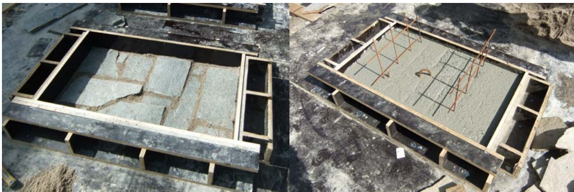
Fig. 3: Stone facing placed into mould (left) and front wall after concreting (right)
