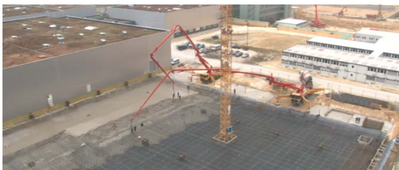
Fig. 5: Casting of foundation raft slab of the Carl Zeiss AG factory in Oberkochen
