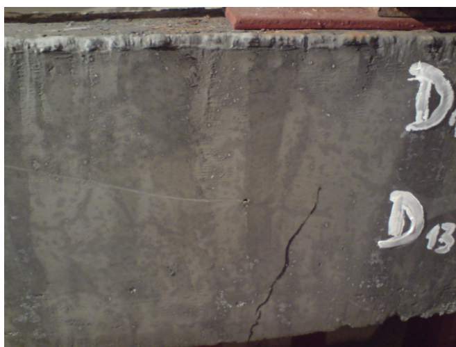
Fig. 5 The appeared of the first crack
