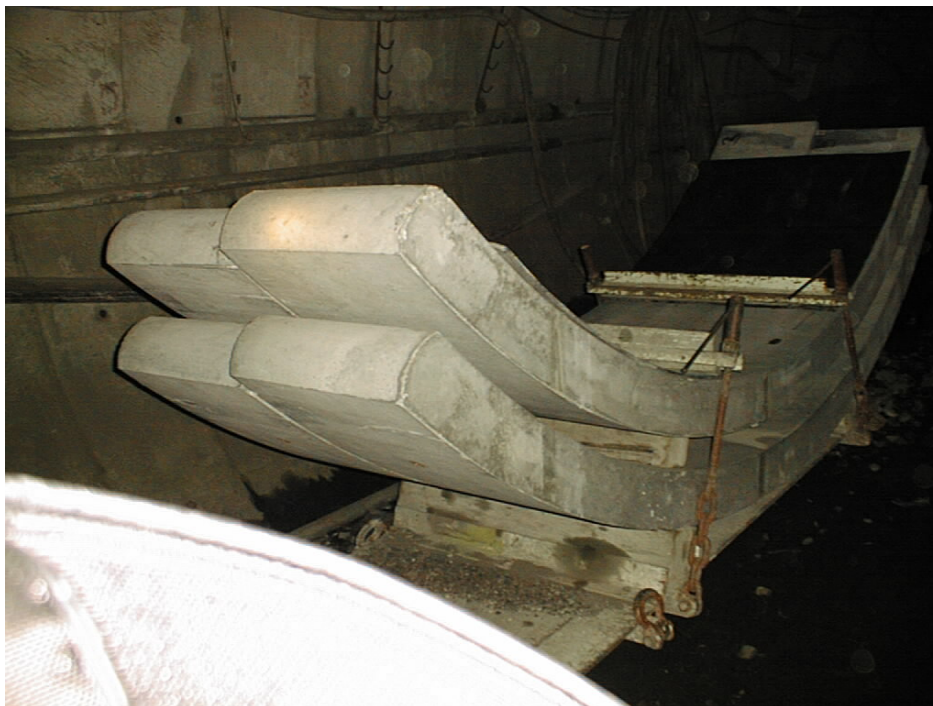
Fig. 15: Panels with HP-FRC ready for installation in the lining of mine roadways.
