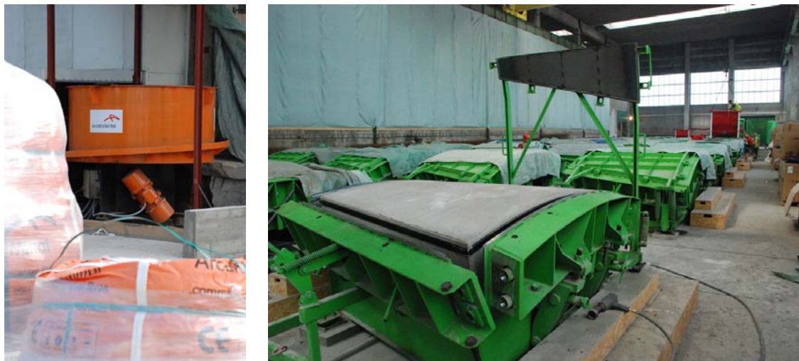
Fig. 1: Steel fibres packed in big bags and an automatic dosing unit (left), formworks (right) – Ejpovice Railway Tunnels
