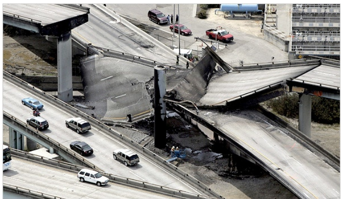
Figure 4: Collapse of I-580 bridge in CA, USA in 2008 as a result of gasoline tanker crash and consequent spillover of the highly flammable liquid (Quiel, Yokoyama, Bregman, Mueller & Marjanishvili 2015). Photo taken from (Jennings & Winton 2011).
