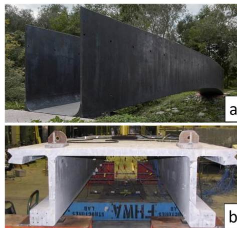
Figure 1: Completed thin-walled UHPC structures: a) footbridge near Vrapice village (KŠ Prefa), b) experimental footbridge with Pi-section (FHWA).
