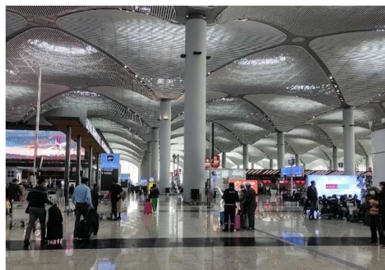
Figure 7: Architectural elements covering the load-bearing structures (Daily Sabah 2022).
