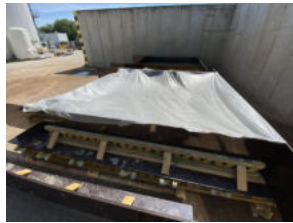
(b) Curing of wall specimens under the plastic foil.
