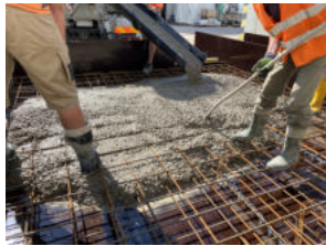
(a) Concreting of reinforced concrete wall specimens.
