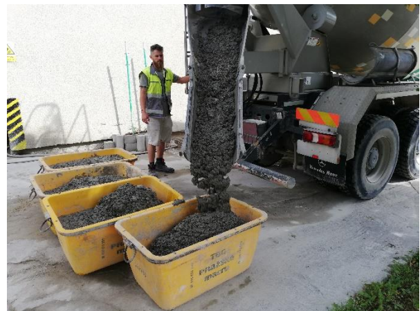
Figure 3 - Execution of experiment at the batching plant [photo: author]
