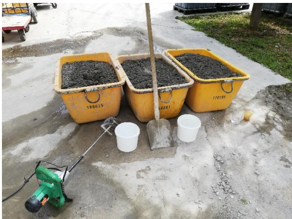
Figure 4 - Three concrete batches before adaption of consistency [photo: author]
