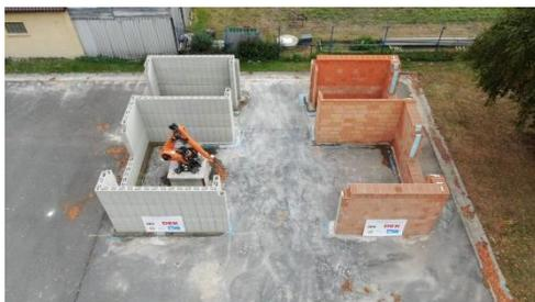
Figure 3: *Dekmatic by DEK in cooperation with CTU*
